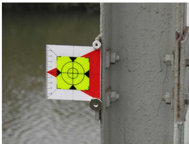
Fig. 5: The measurement targets (on magnets) were temporarily installed.
