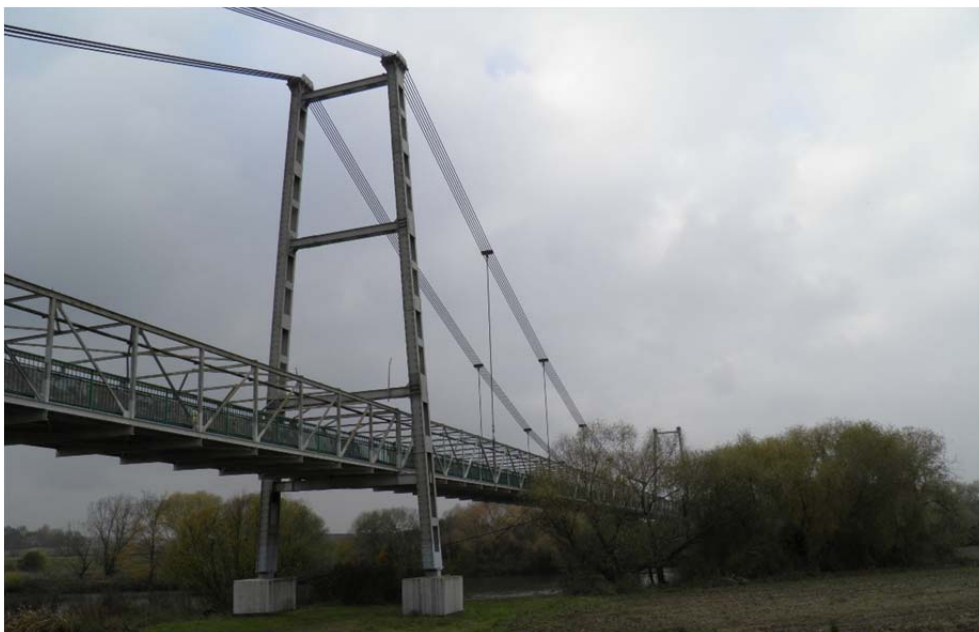
Fig. 2: The pylon of the bridge.
