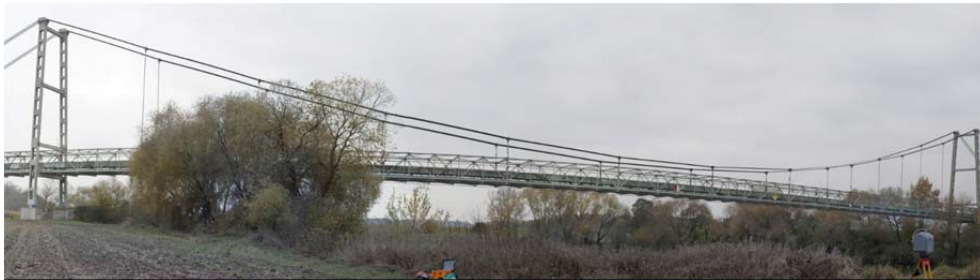
Fig. 1: View of the bridge from the upper water side.
