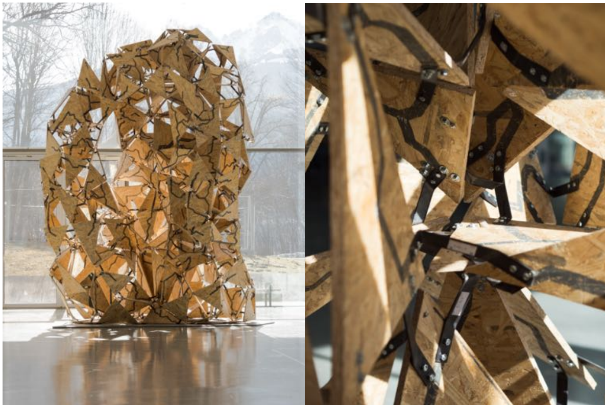
Fig.11 the final tower and a detail of the joints with generated pattern
