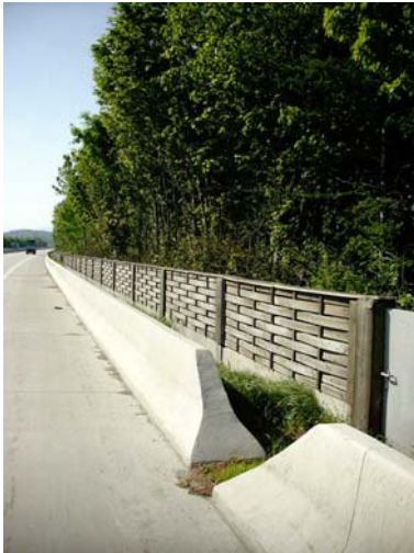
Fig. 4: the formerly existing noise wall
