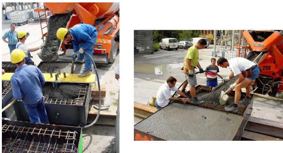
Fig. 3. Casting of large-scale specimens for fire experiments under on-site conditions [10].
