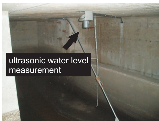
Figure 3.7: Water level measurement in Innsbruck - Water level measurement in Innsbruck via ultrasonic device
