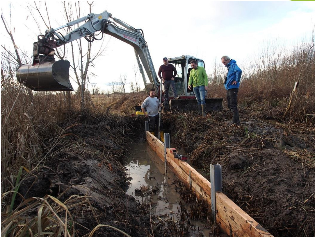
Ditch construction, photo: G. Käfel
