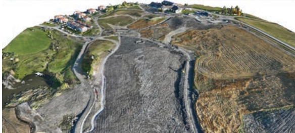
Figure 2: The northern part of the landslide area.
