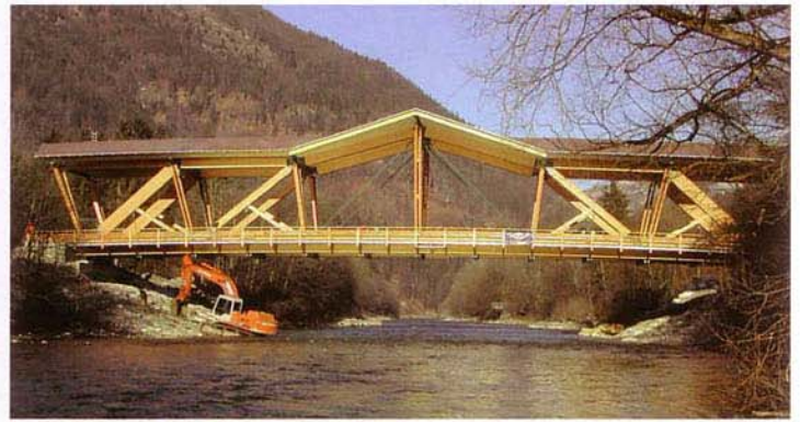
Kossen road bridge, Germany Structural Engineer: Michael Flach, University of Innsbruck Photo courtesy Michael Flach
