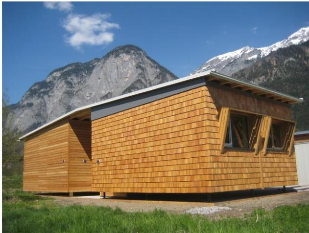
**Figure 3:** Realized wooden building modules from the outside (left: CLT-construction, right: wood frame and clay construction)
