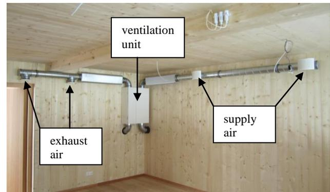
**Figure 1:** built in mechanical ventilation system in the wooden module
