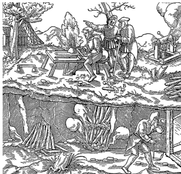
Fig. 3 Fire-setting as depicted by Georgius Agricola in his De re metallica libri XII from 1549 (Schiffner 1928). A burning pile of wood, B Bärte (frayed pieces of wood for kindling fire), C mine shaft
