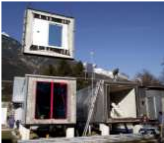
View of both test cells and replacement of one test facade
