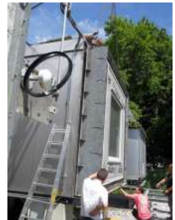
Mounting of test component (Project water:solution)
