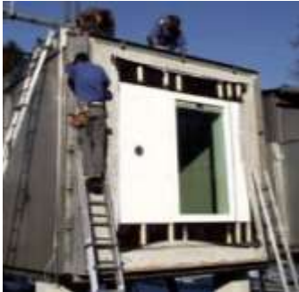
Mounting of test component (Project INTENSYS)
