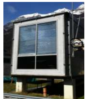
Outside view test component with complex façade system (Project K-Licht)
