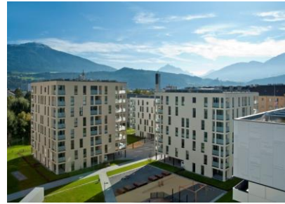
Innsbruck Passivhouses O3 with solar thermal plants
