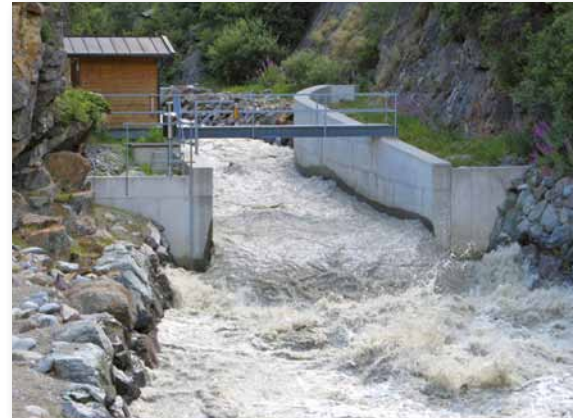
The water gauge 'Vent/Rofenache'; Measurements comprise water level (with RADAR and a pressure probe), surface flow velocity (with RADAR), water temperature, suspended sediments (with a turbidity probe), and bedload (with a geophone). All data are measured continuously, recorded on site and transmitted via GPRS (photo: Hydrographical Service Tyrol)
